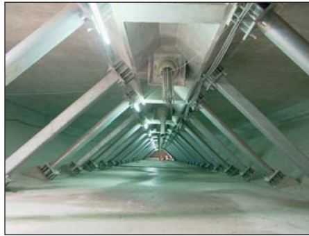
Fig. 5: Steel pipe bracing
