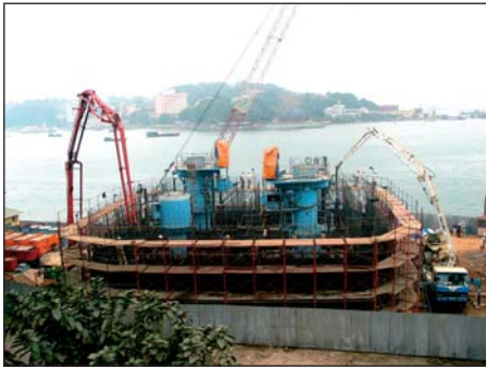
Fig. 3: Pneumatic caisson foundation
