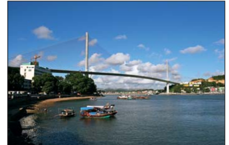
Fig. 1: Bai Chay Bridge
