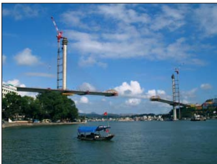
Fig. 4: Cantilever erection
